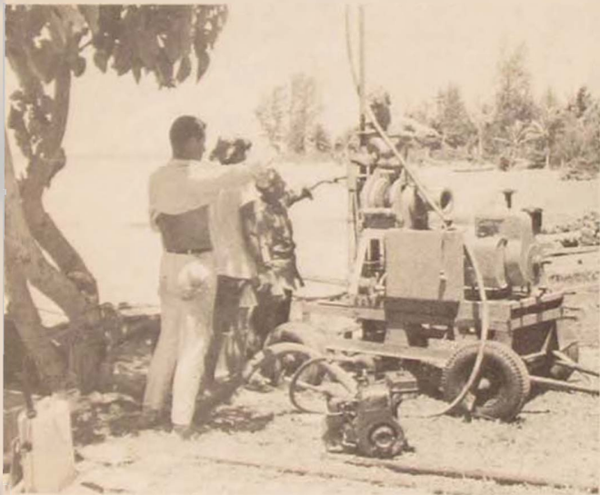
Somewhere in Korea, a site selection team orients a map to the local terrain, using a plane table . . . prepares to drill 50 feet for subsurface exploration.
